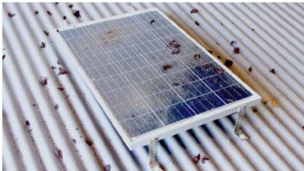
If solar panel is dirty...
